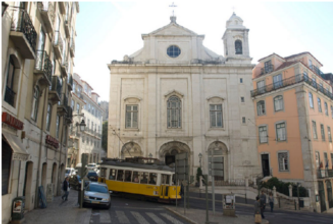
Fig. 9) Founded in the 12 th century by order of the first Portuguese King, Afonso Henriques (r. 1143–1185), shortly after the conquest of Lisbon from the moors. The Magdalena Church underwent many alterations and reconstructions over the centuries. The current temple was inaugurated in 1783 and reflects a sobriety characteristic of the Pombaline reconstruction and the use of ancient elements.
